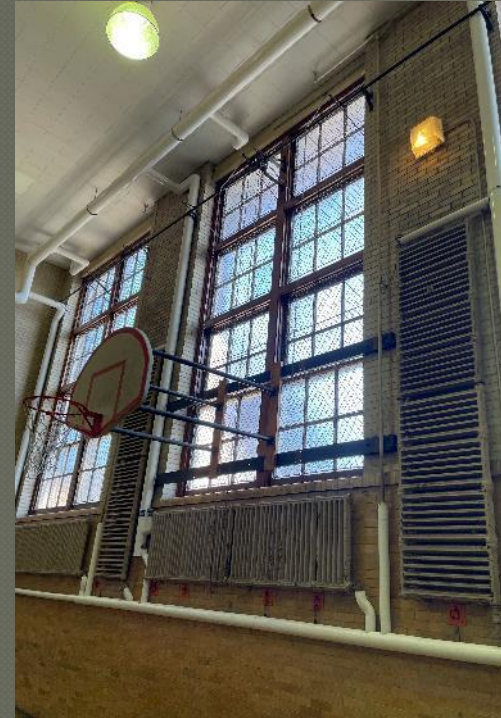
Interior view gym windows
