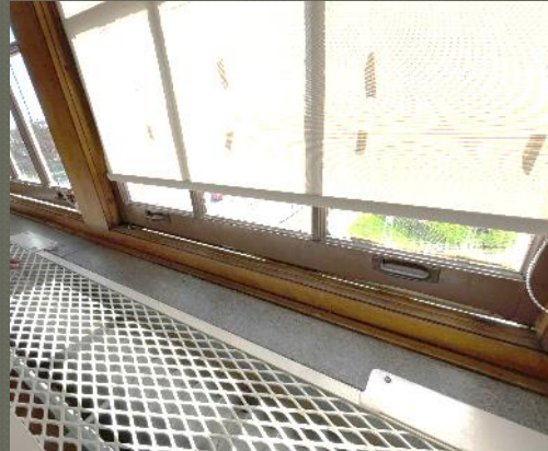
Interior view existing window
