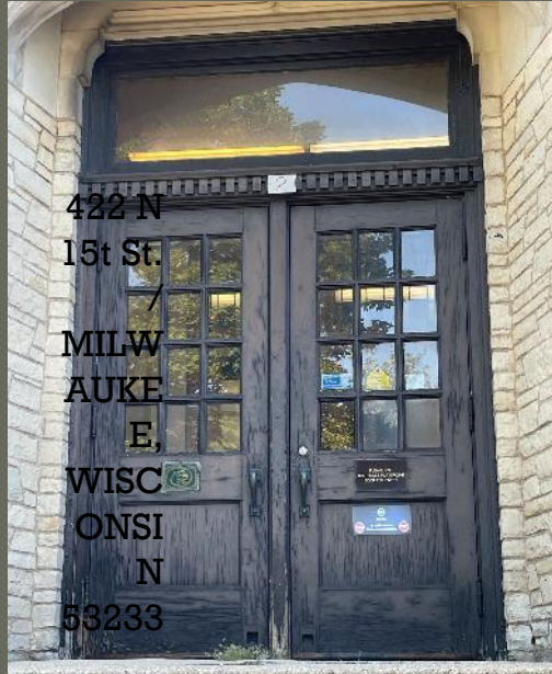
Existing entry doorway
