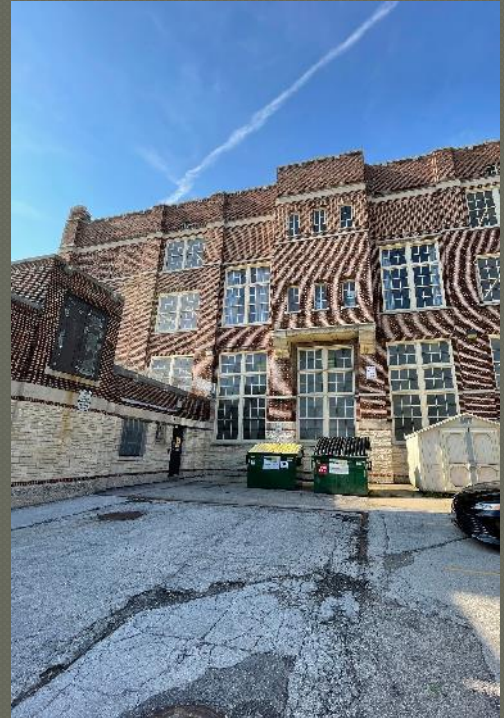
North elevation exterior view
