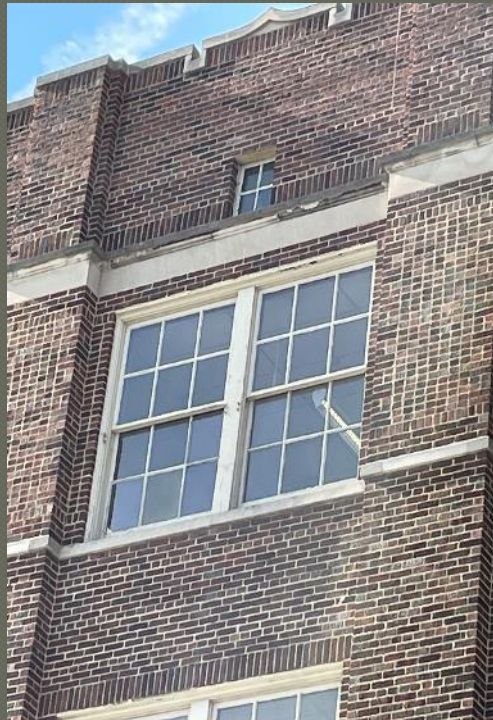
View of exterior existing window
