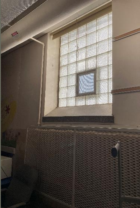
Interior view glass block window
