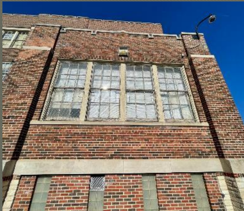
View of exterior existing window
