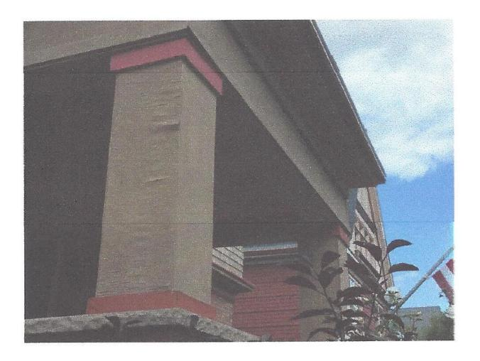
Front porch columns to be reconstructed in new wood. Capitals must match details from porte cochere columns shown on next page. Base must be complimentary to capital design and feature molded details.
