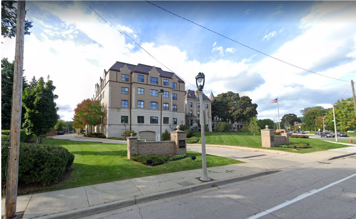
Watertower – Southeast View from Lake Dr public way
