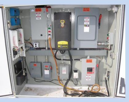
Sanitary Bypass Pump Controls
