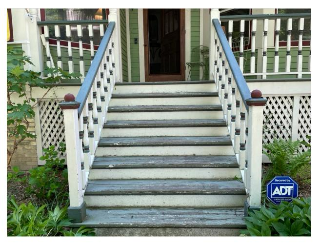
Option 1 is like for like replacement of wood stair elements—treads, risers, railings and spindles—as needed
