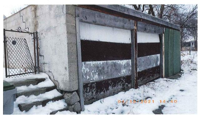
Violation 14. Repair defective blocks in exterior wall of the garage.
