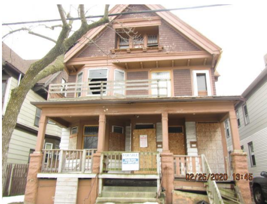
Above: 629-31 West Clarke Street
