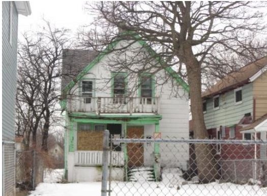
Above: 2421 North 6th Street
