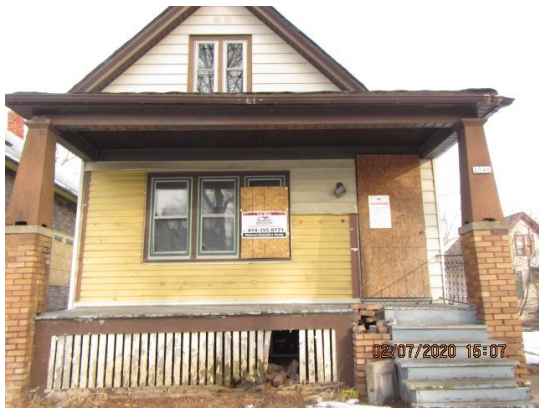
Above: 2946 North 6th Street
