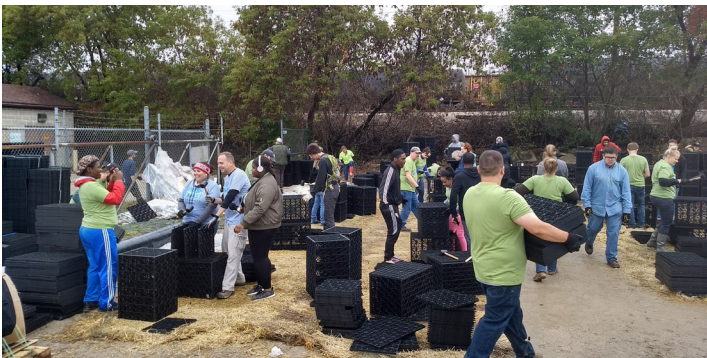
More than 90 volunteers helped assemble aqua blox that make up the 20,000 gallon underground cistern at Green Tech Station in October 2018; cr. NWSCDC
