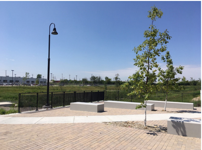
Permeable pavement plaza space and seating area at the northeast corner of the North Basin; cr. MMSD
