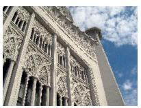
**Figure 4**. The highly ornamental concrete panels on the exterior facade of the Baha'i House of Worship in Wilmette, Illinois, illustrate the work of fabricator John J. Earley, known as "the man who made concrete beautiful."
