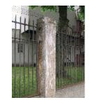
Figure 15. Evidence of moisture movement through concrete is apparent in the form of mineral deposits on the concrete surface. Cyclic freezing and thawing of entrapped moisture, and corrosion of embedded reinforcement, have also contributed to deterioration of the concrete column on this fence at Crocker Field in Fitchburg, Massachusetts, designed by the Olmsted Brothers.
