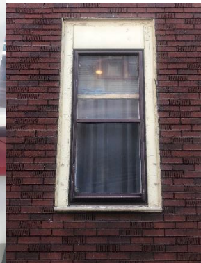
Typical existing conditions and typical existing storm window.
