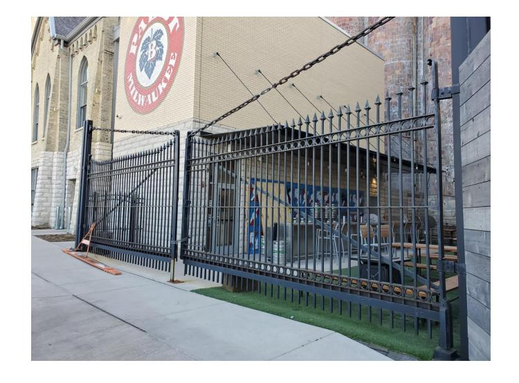
CCF 160575 1037 West Juneau Avenue 3-17-2020 Looking northeast from North 11<sup>th</sup> Street at the gate. The north leaf is locked in place, while the south leaf can swing open over the sidewalk and into the roadway.
