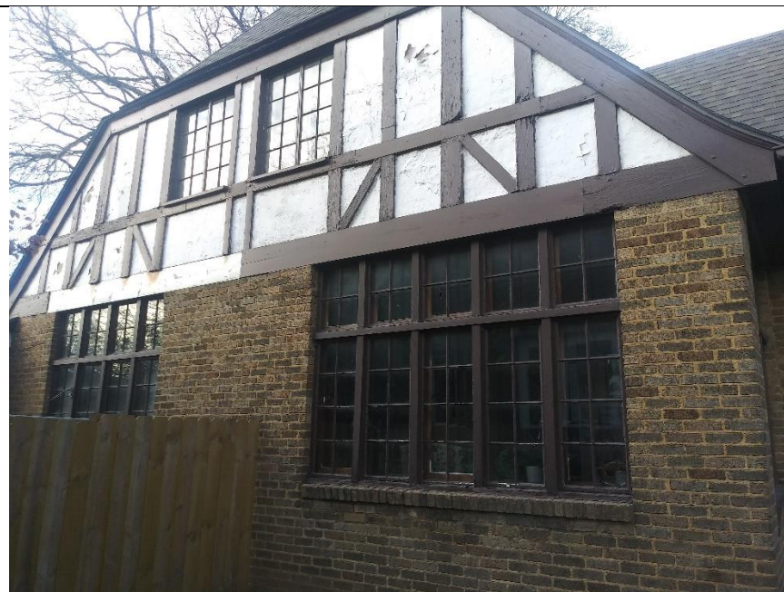
South elevation showing typical state of stucco and siding
