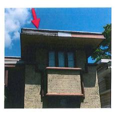
(Bid Package #1) Order to Correct #5 Replace defective trim boards on exterior walls (SOUTH SIDE MULTIPLE AREAS)
