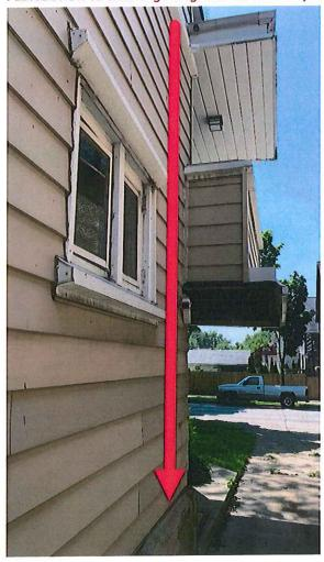
(Bid Package #1) Order to Correct #10: Replace defective facia boards (WEST SIDE)
