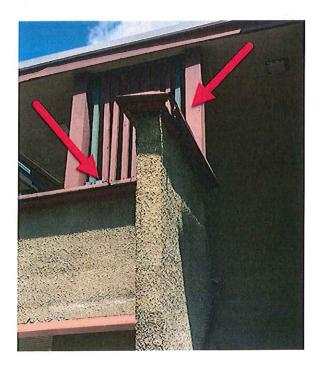
(Bid Package #2) Order to Correct #6 Repair or replace defective handrail on porch steps
