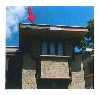
(Bid Package #1) Order to Correct #5 Replace defective trim boards on exterior walls (SOUTH SIDE MULTIPLE AREAS)
