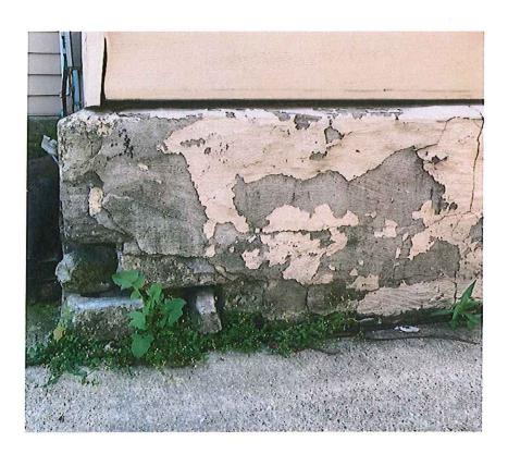
1.2. Order to Correct #12: Replace defective blocks in foundation wall - NORTH
