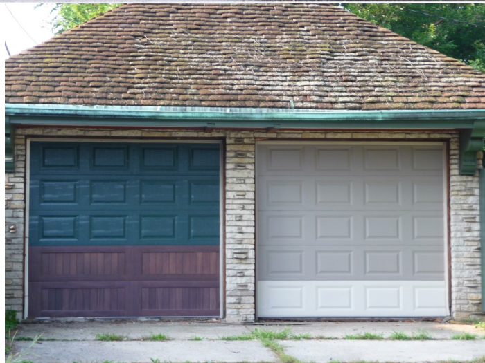
"Temporary" doors as of late August 2018.
