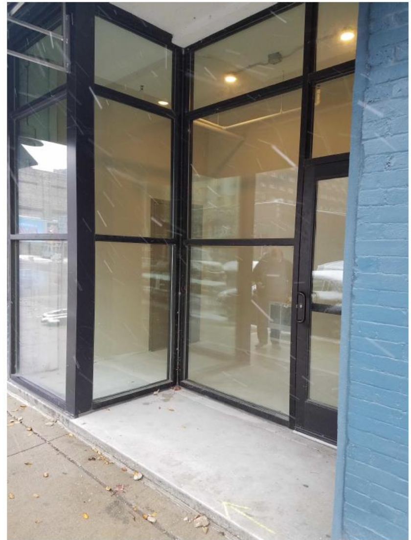
EXTERIOR VIEW LOOKING @ ENTRY
