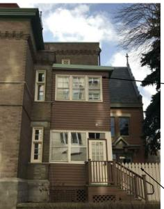
DORMER ORNAMENTAL METAL WORK TO BE REPLACED TO MATCH EXISTING WITH MISSING THIS WORK WILL MATCH THE PREVIOUS ORNAMENTAL METAL WORK PLACED ON REST OF FACADES. WINDOW IN DORME TO HAVE REPLACEMENT SASH WITH 1/2" INSULTATE GL
