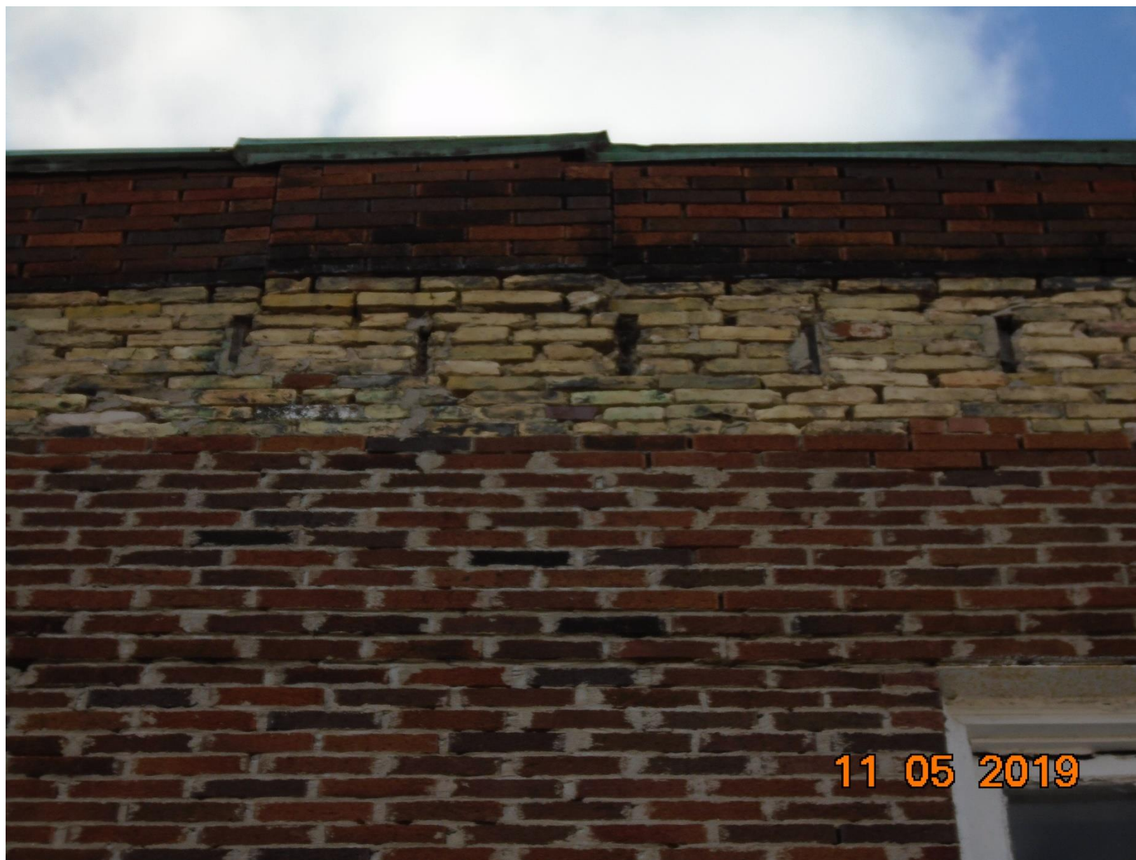
Detail of damaged area. Note subtle pilasters and copper coping. Pilasters and copper coping will be required in the reconstruction.
