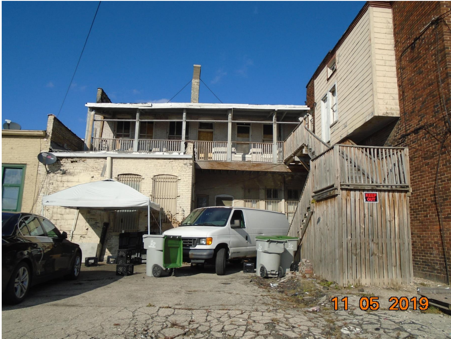
Rear of 705-707 building. Porch roof and all chimneys are to be removed. Porch over the rear bumpout (with bars on windows) shall be demolished, but columns and corbels shall be retained for reuse.
