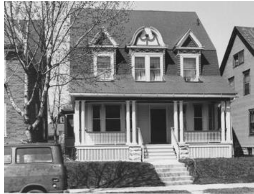
Porch measures 31 feet wide by 7 feet deep. Railing is 29 inches high. Skirting boards are 1" by 8" frame and 1" by 6" verticals.
