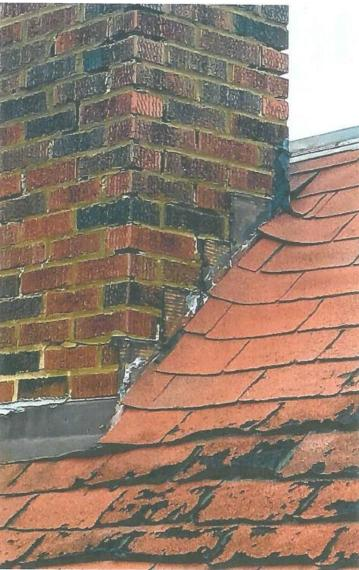
Chimney to be step flashed (as is shown in the present condition above) and repointed with appropriate mortar, as close as possible to **US Heritage Group color SC Sahara (2)**
