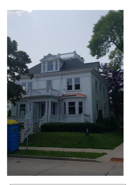
Porch roof and widow's walk will have new membrane roofs. Bays will have roofs with copper cladding.
