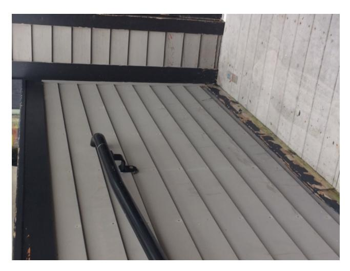
Existing landing area for ADA access to restaurant. Opening to be made to deck at landing, beyond existing hand rail. Deck to be level with landing.
