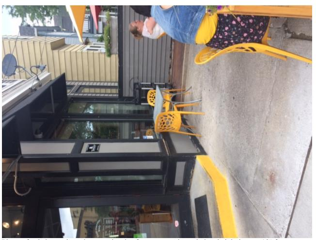
Photo of existing patio and uneven levels of concrete. Also, window height is over 18" from existing patio.
