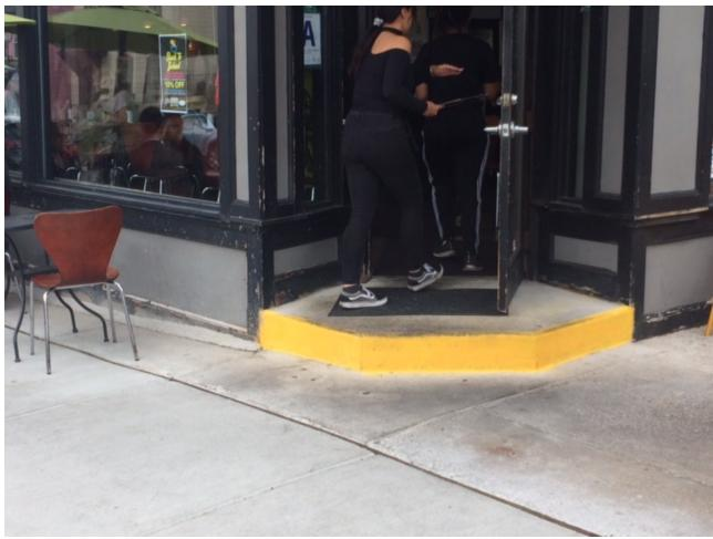
Existing front step, 7" h. Deck to continue at that level to right of main entry.
