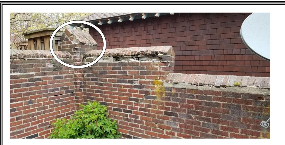
Posts must be rebuilt only with new brick. Limestone caps are not permitted.
