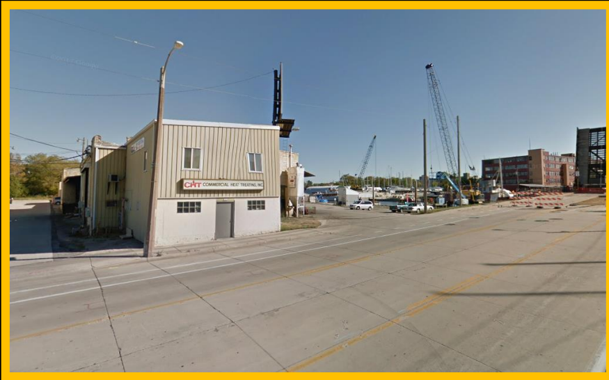
View from East Anderson Ave and South 1 st Street
