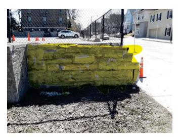
Reconstruct Highlighted Area With Integrity Masonry Units Proposed
