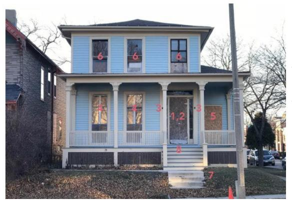
The door numbered 5, at right, will be replaced with the wood window shown on the following page. New trim shall match existing window trim on the house.
