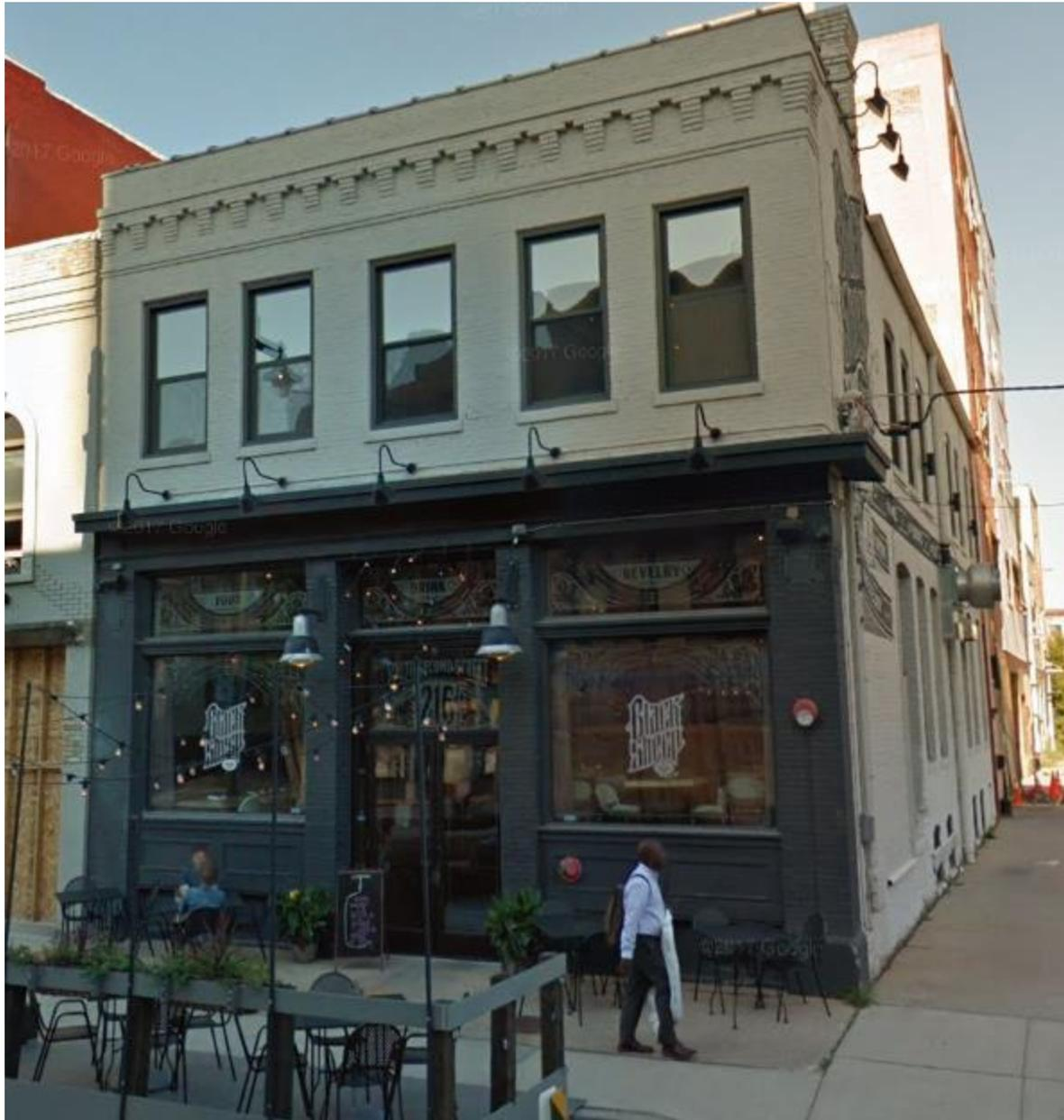
**Must retain terra cotta coping or install replicas on front (west) elevation pictured here.**
