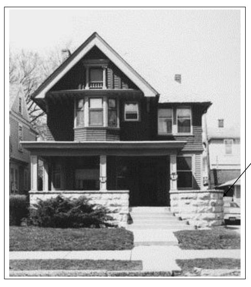
Front porch will be carefully deconstructed and rebuilt using the same stone. The stone walls are five courses high with an interior of brick.
