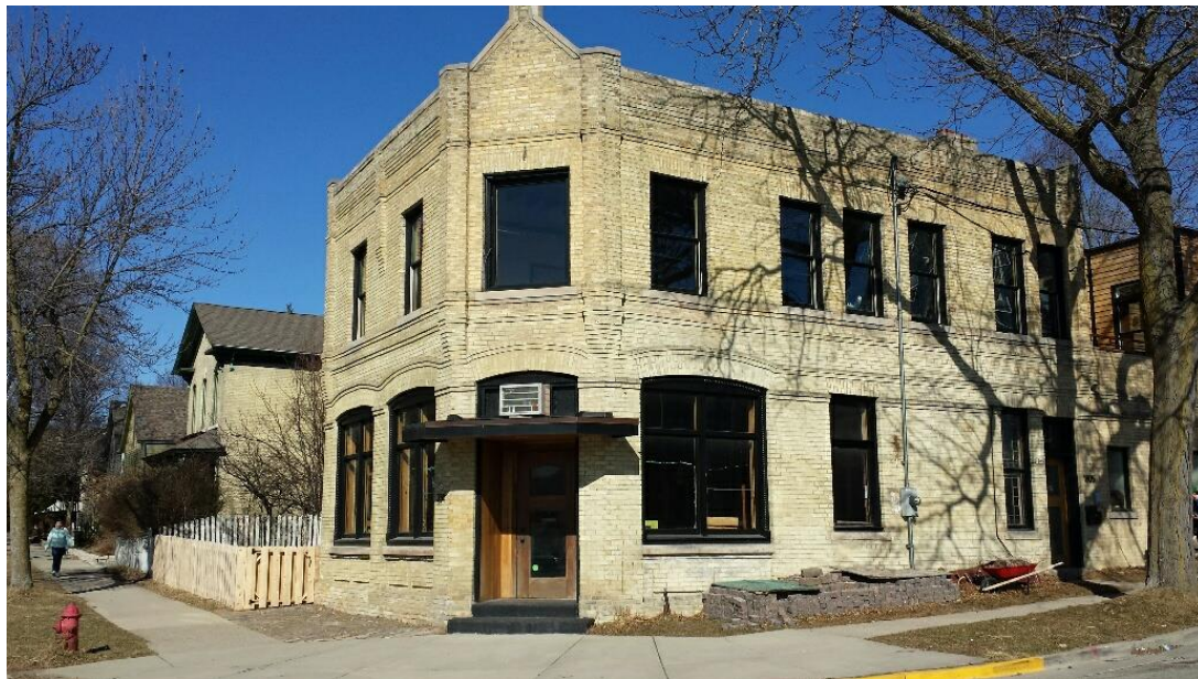
Looking northwest at main entrance.
