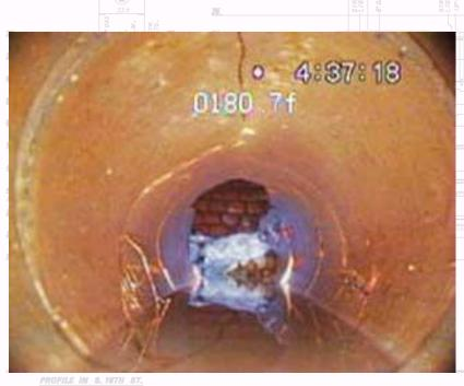
Before – Sewer is cracked and deteriorated. Water from the ground can enter the sewer freely. After – Sewer is smooth and sealed. Water from the ground can no longer enter the sewer.
