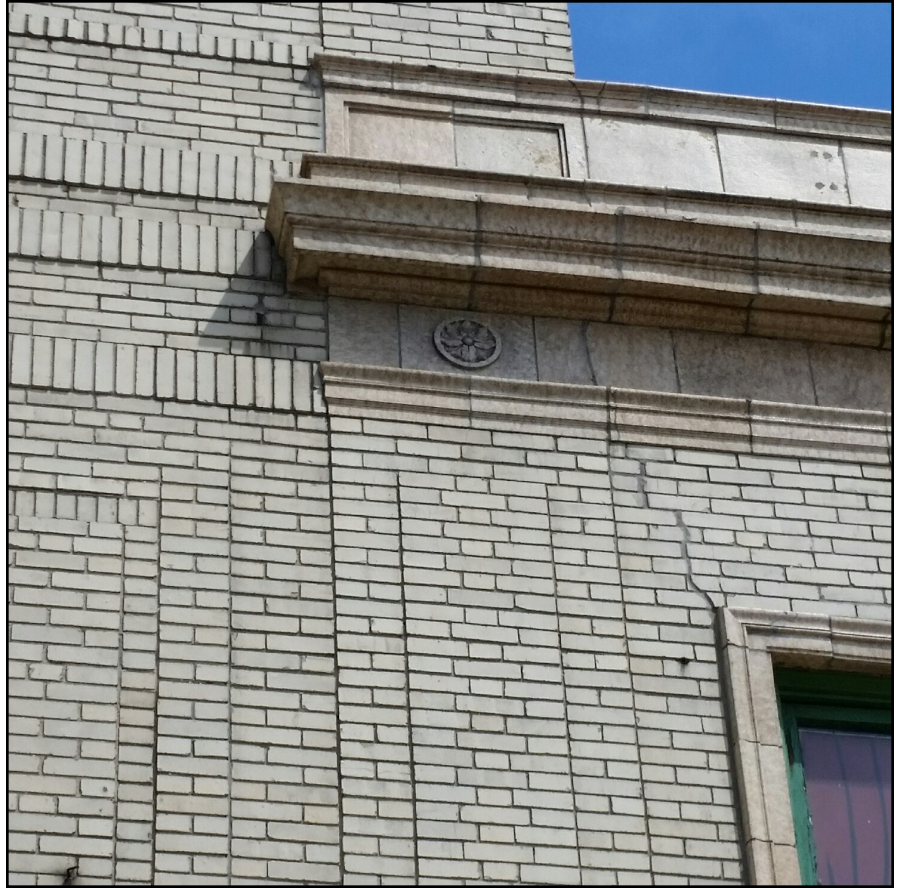
Close up and Distant view of Cornice and brick repairs on West face of build- ing at second floor.
