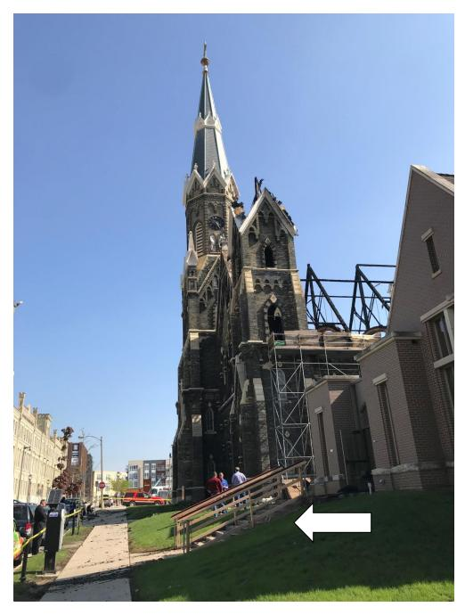
Replace temporary railing with new metal one to match original. Cut and patch concrete as needed.
