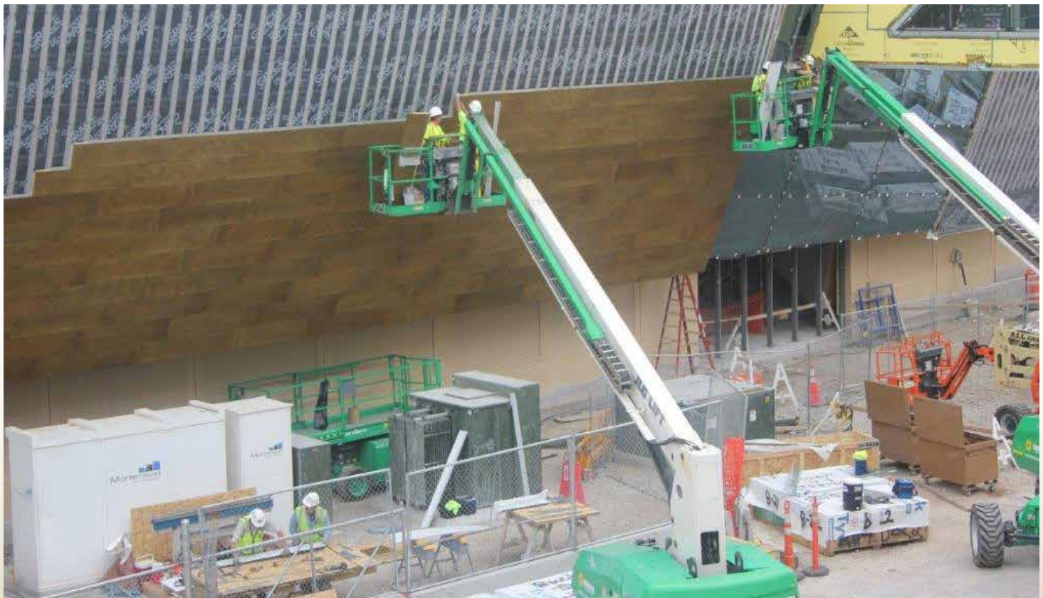
Sheet metal workers installing façade on the WESC
