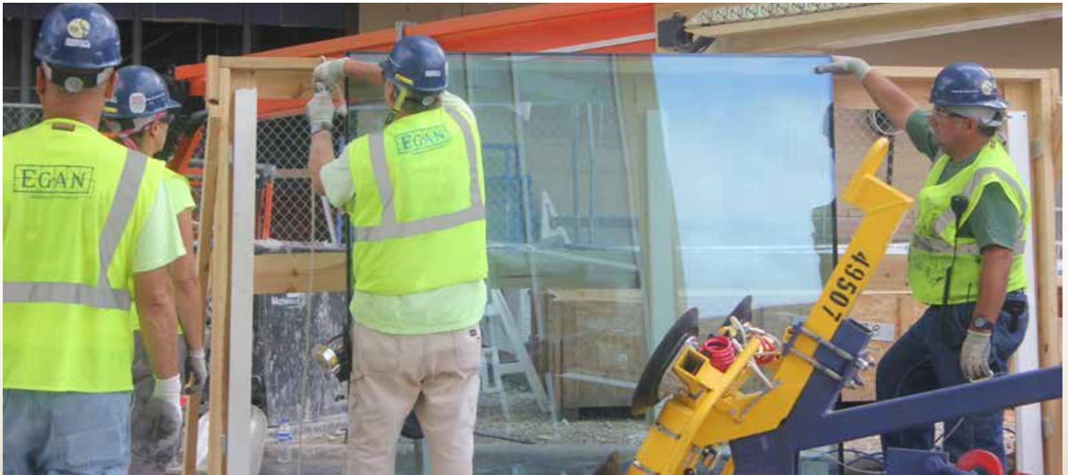
Workers installing glass panes on 5th Street Parking Structure.
