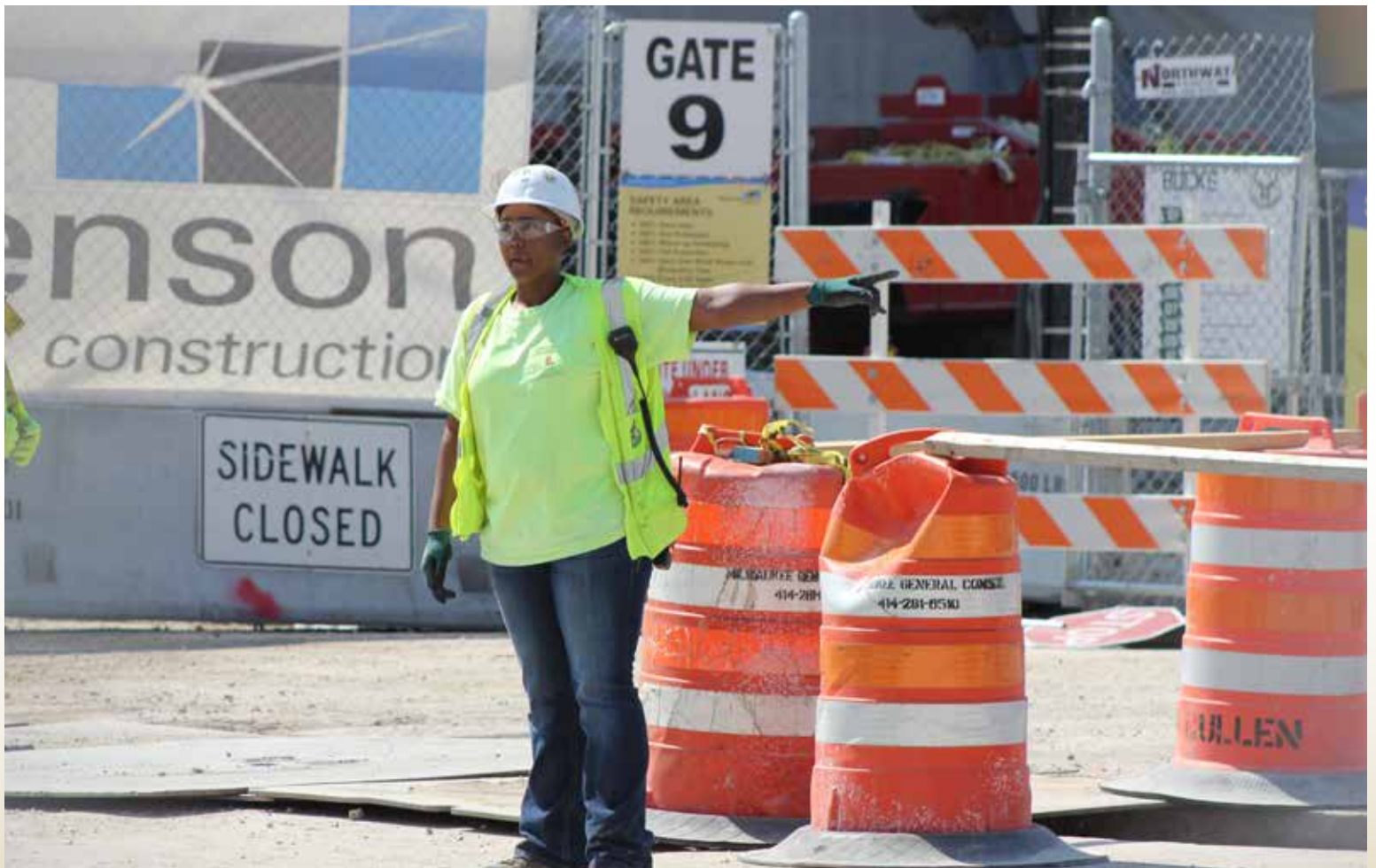
Worker directing traffic on the WESC construction site.
