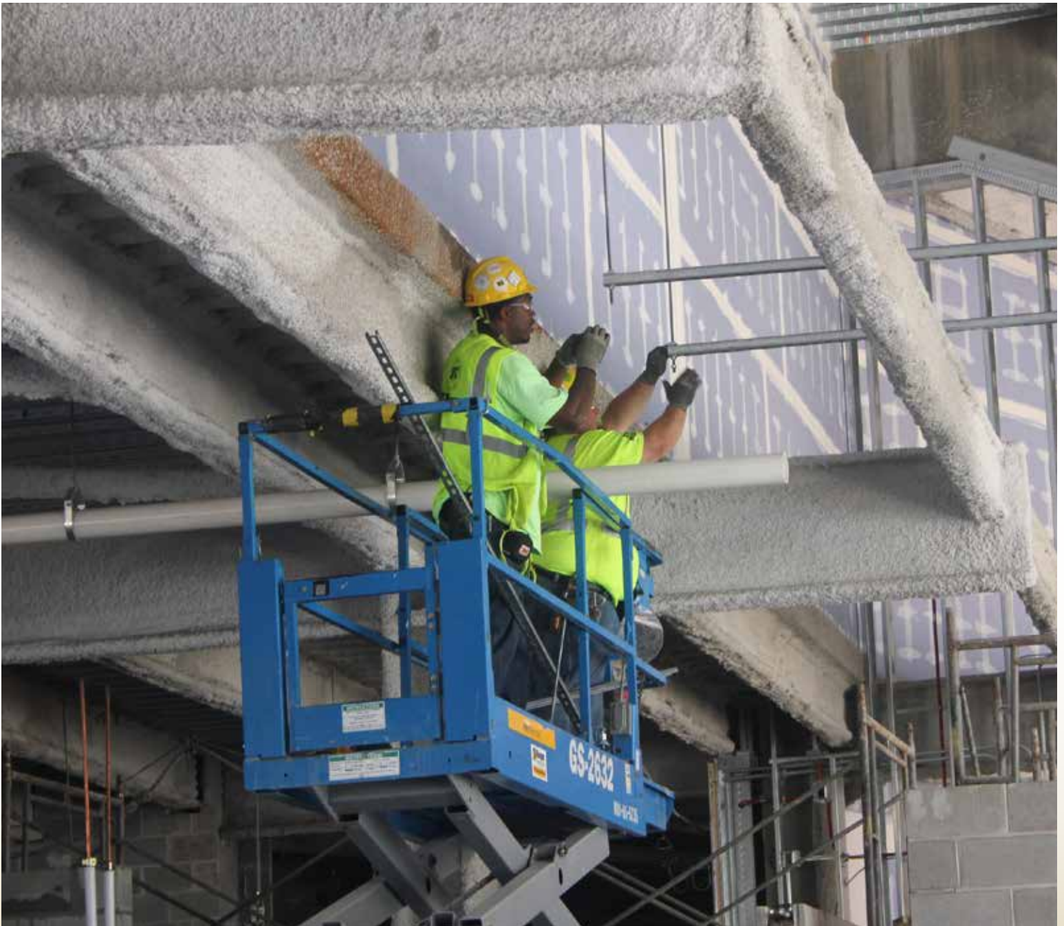
Workers on WESC construction site.
