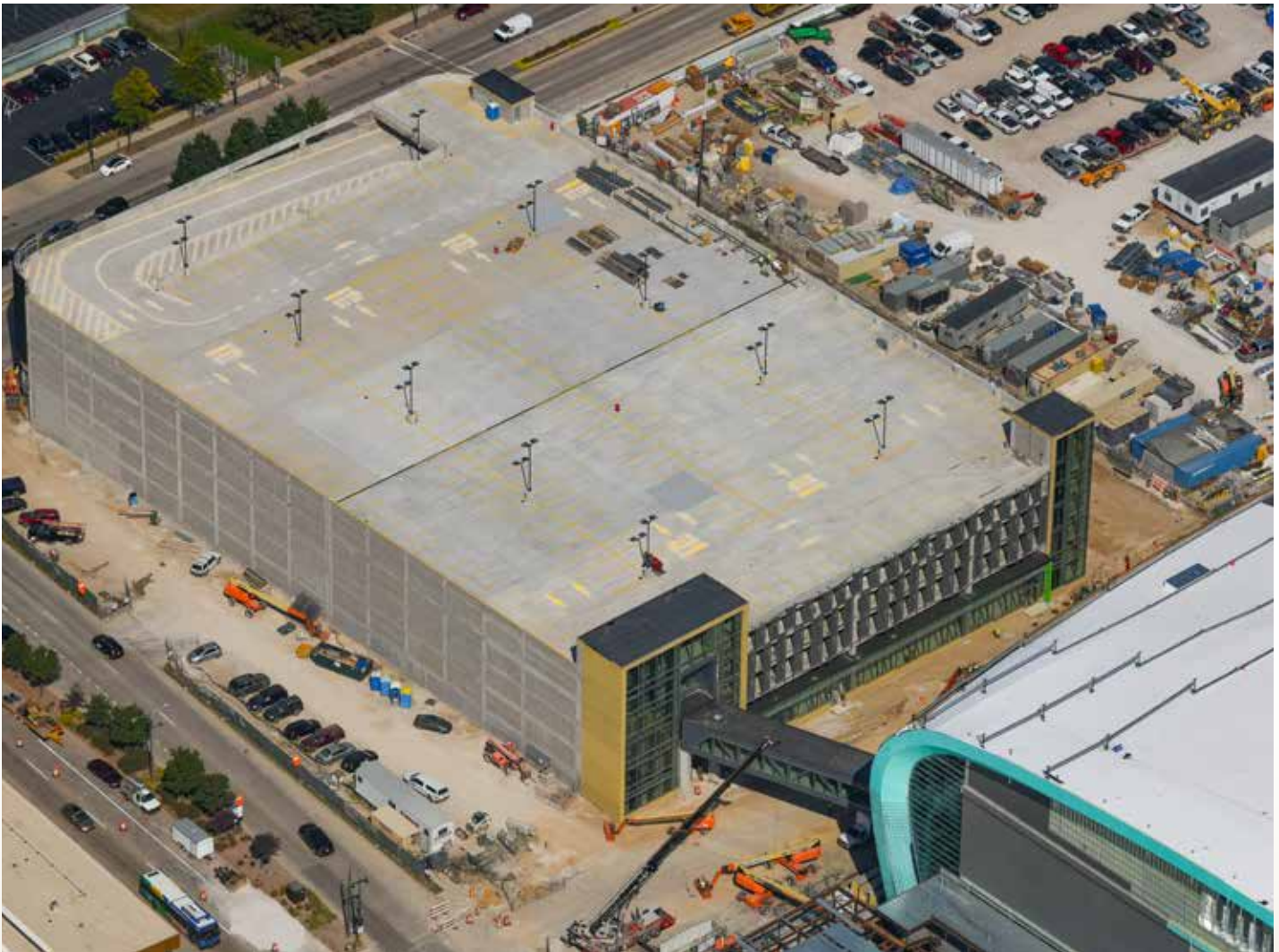
Aerial view of the WESC and 5th Street Parking Structure - September 2017.
