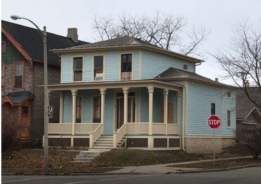
EXISTING HOME IN CURRENT STATE 2017 (photo credit: a. raabe)
