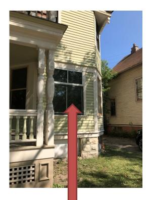
The large landscape sash at the front of the house (west elevation) will be returned to its original condition with one large pane of glass below the fixed transom window. The bottom storm window on the exterior can remain with two panes of glass.
