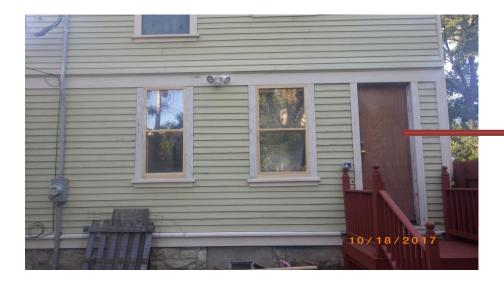
The rear door will be painted and a wood storm door installed. The wood storm door will also be painted.
