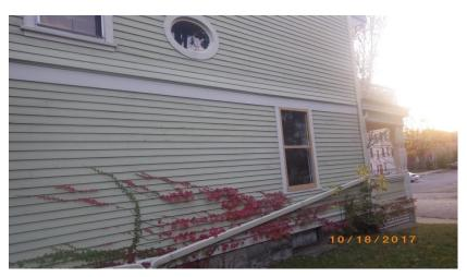
Vines will be removed from the north side of the house. They can do considerable damage as they work their way under the clapboards.
