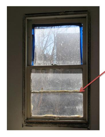
This window, located on the second story of the south elevation facing the driveway, can remain. The bottom sash is divided into two panes.
