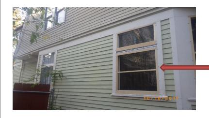
This window is located on the south elevation and faces the driveway. The bottom sash can remain divided into two panes. The wood storm on the bottom portion of the sash can remain divided into two panes. The storms must be painted.
