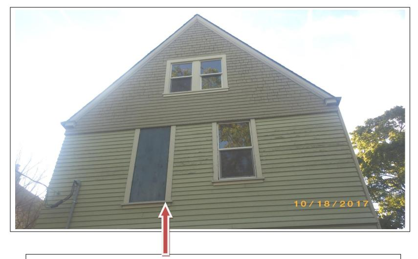
Jump porch has been removed. Door that accessed platform is being removed. Plywood will fill the opening and the trim will be removed. Wood clapboard siding to match existing will be installed, and will be staggered to blend in with the existing wood siding.
