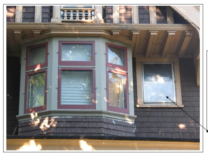
This window appears to have been added after World War II. It will be removed. The resulting opening will be sheathed over with wood shingles that match the existing and have the same exposure.
