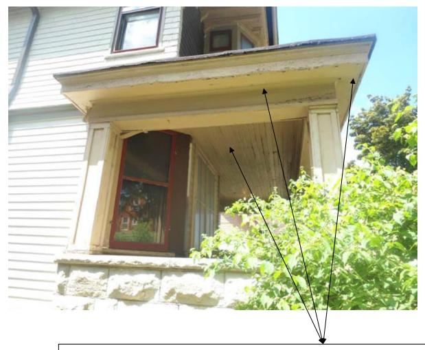
Replacement porch roof will have the same features as the current one with overhangs, appropriate molding profiles and beadboard/tongue-in-groove ceiling.
