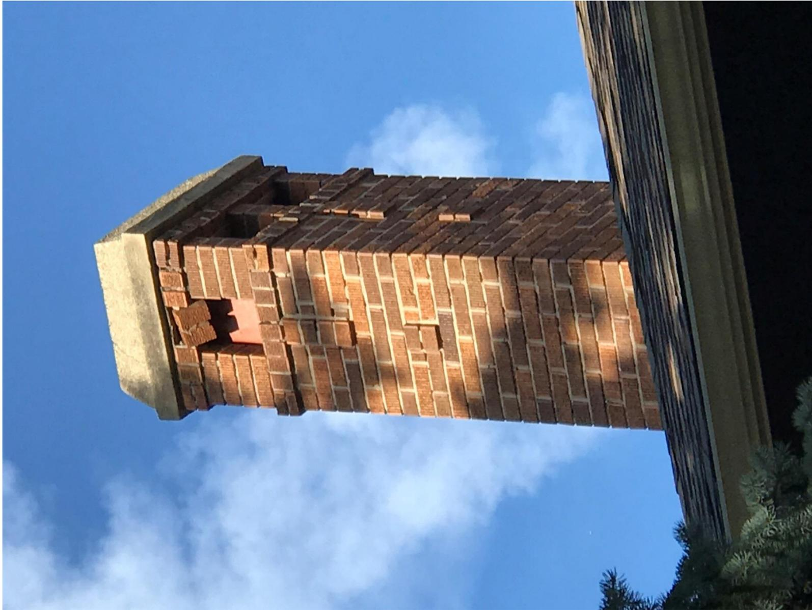
Chimney with failing bricks to be repaired. Because of the position of these brick, type N mortar may be used, but O is preferred if feasible.
