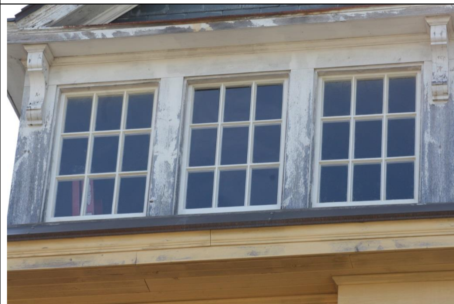
Replacement windows as installed.
