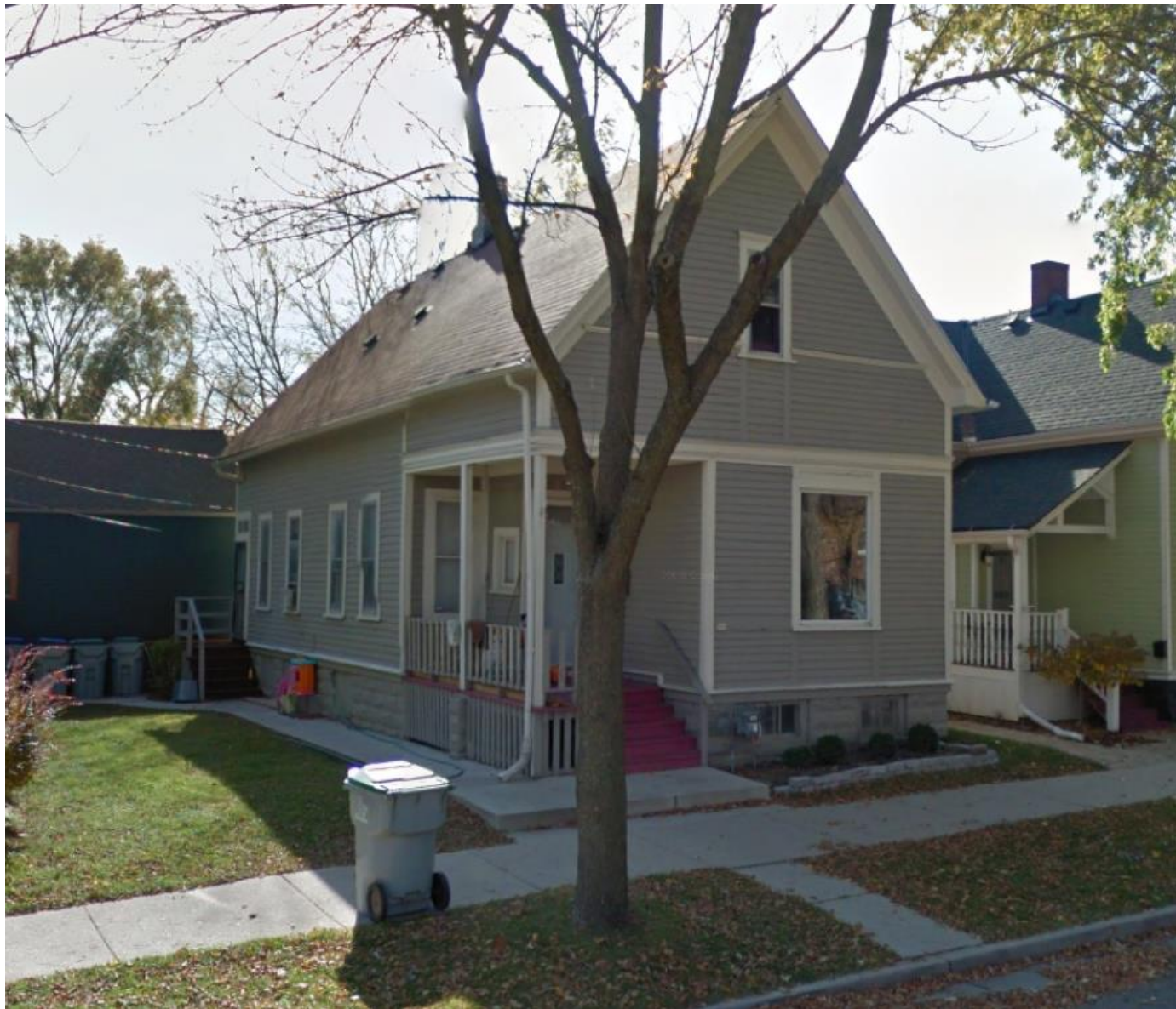
Fall 2015 view from Google. Porch railing is to be replaced and extended to the sidewalk. Spacing of boards in skirting is to be tightened.
