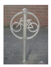
Bicycle racks that lack any point of frame contact are not allowed, and existing 1-point of contact racks may continue to be counted as compliant bike parking space.
