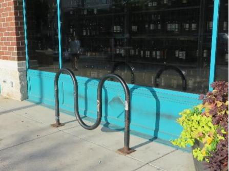
While an acceptable U-Rack, it is mounted too close to immobile planter to allow bike to positioned next to it.
