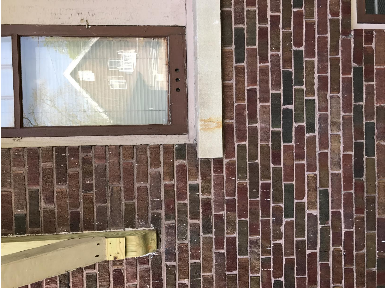
Mortar color to match is immediately left of window.
