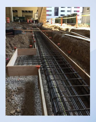
OCS Pole foundation and footing excavation and construction ongoing
