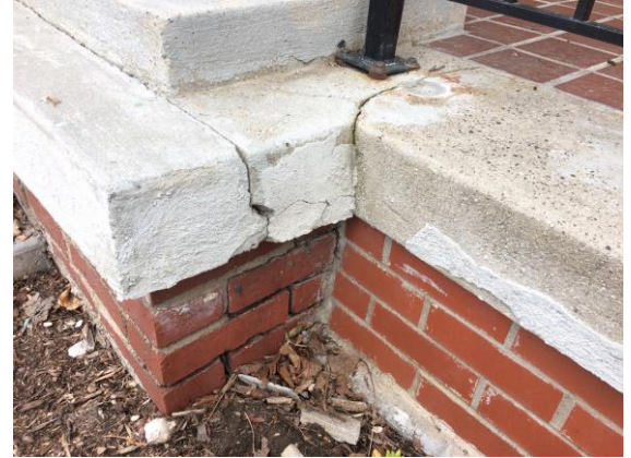
Close ups of old and new brick facing, failing patched concrete, and
