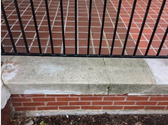
Close up of seam between old and new concrete crumbling mortar
