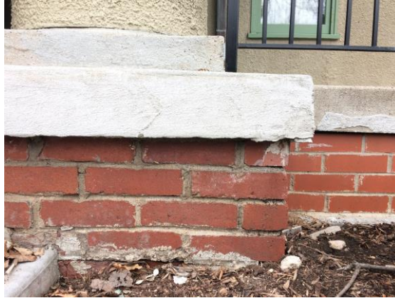
Close ups of old and new brick facing, failing patched concrete, and
