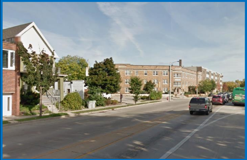
View from West Lisbon Avenue, looking east
