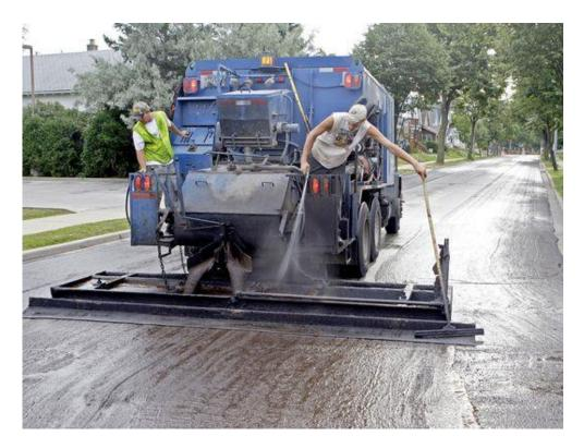
Mike Daffison, left, and Micah Jacobson of Struck and Irwin Paving, apply slurry seal Aug. 12, 2011, to East Bennett Avenue in Milwaukee's south side. (Photo: John Klein, Milwaukee Journal Sentinel)
