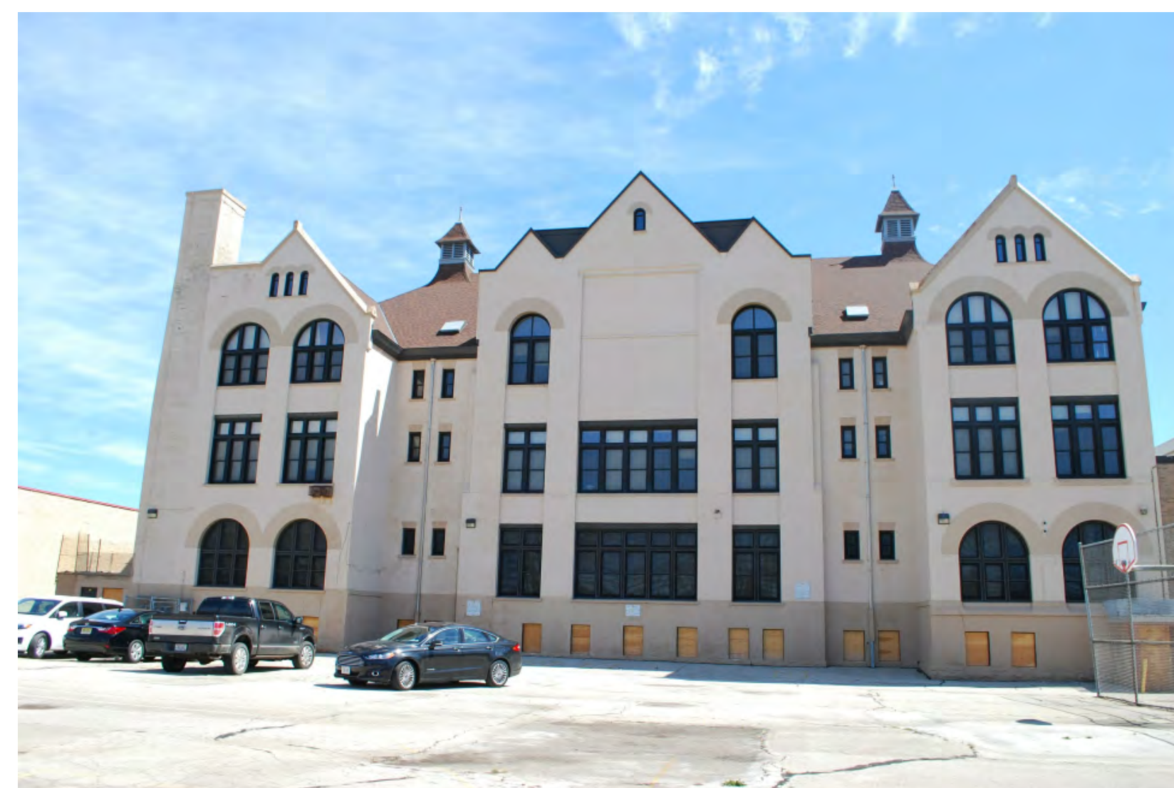
5 - SCHOOL - WEST FASCADE
