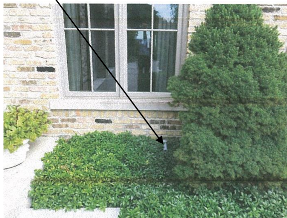
Existing discharge pipe for the back up sump pump. Elbow would be attached at the end to raise the pipe up three inches and extend it out 13 additional inches. This would comply with code.
