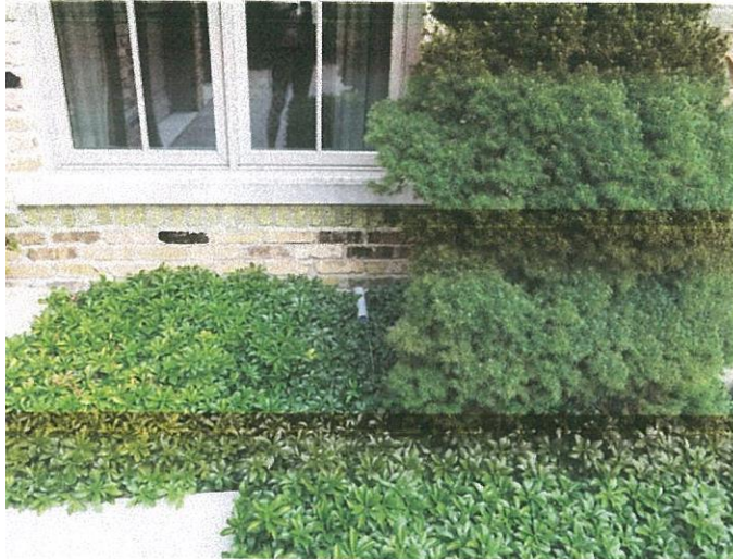
Pipe with slim wire protruding to indicate the additional length need to comply with code.
