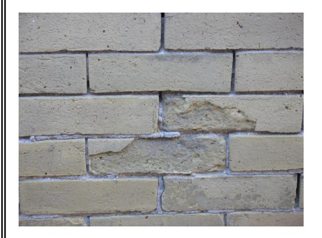
Example of deterioration caused by the use of Portland cement instead of lime-based mortar on another historic property.
