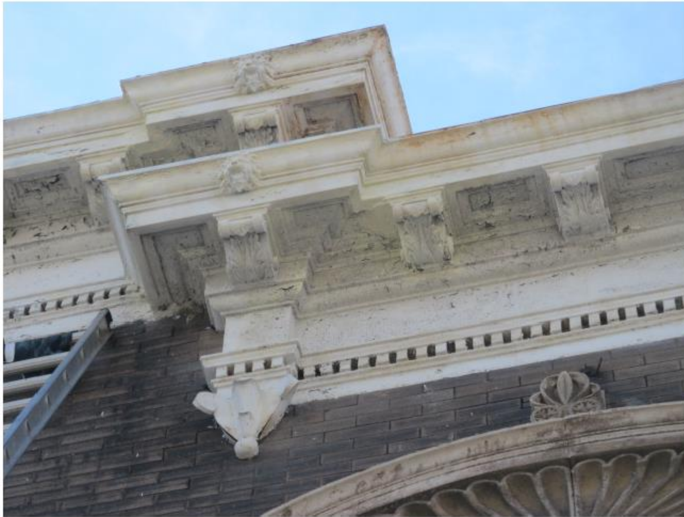
Upper Cornice – repaired with formed sheet metal
