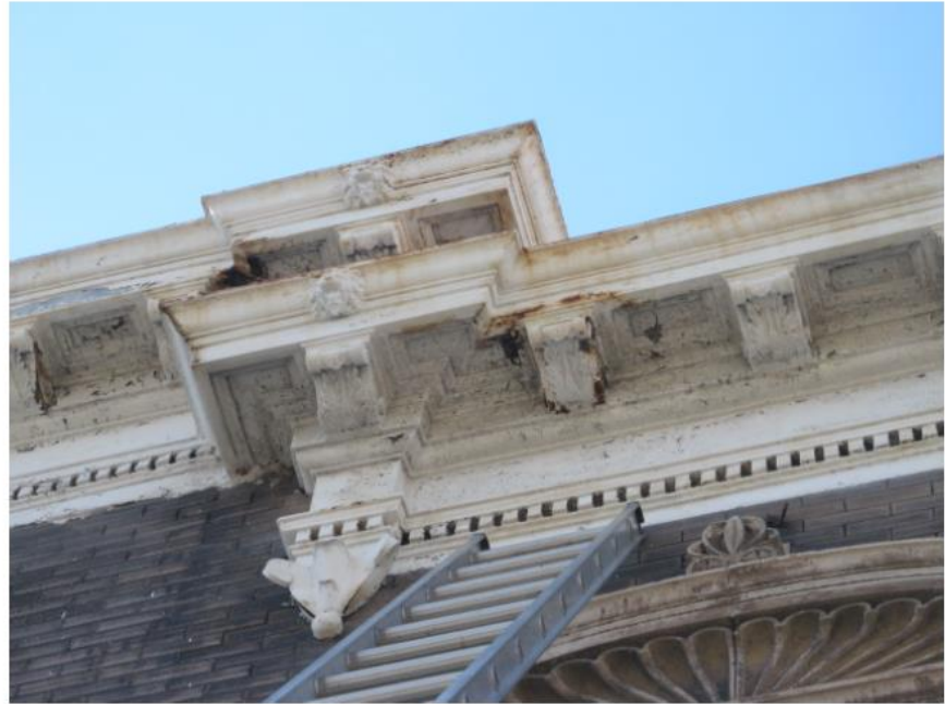
Upper Cornice – rusted holes in metal
